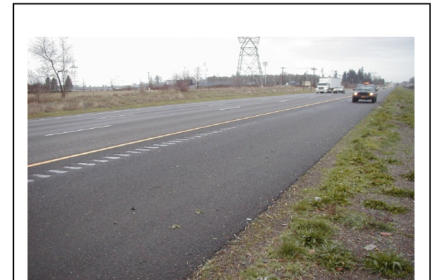
Shoulder rumble strips, like the one above, help save lives.
