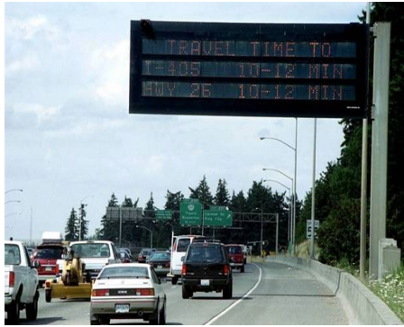
Variable Message Signs convey road conditions to travelers
