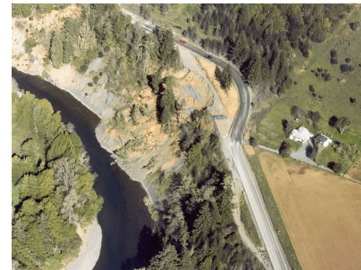
The Powers Landslide at Mile Post 14
